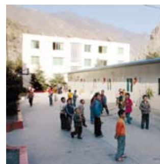
At the end of 2009, 263 school children and 28 teachers from Taoping, China, were able to move into their renovated school. Their old school was destroyed by an earthquake in 2008.
